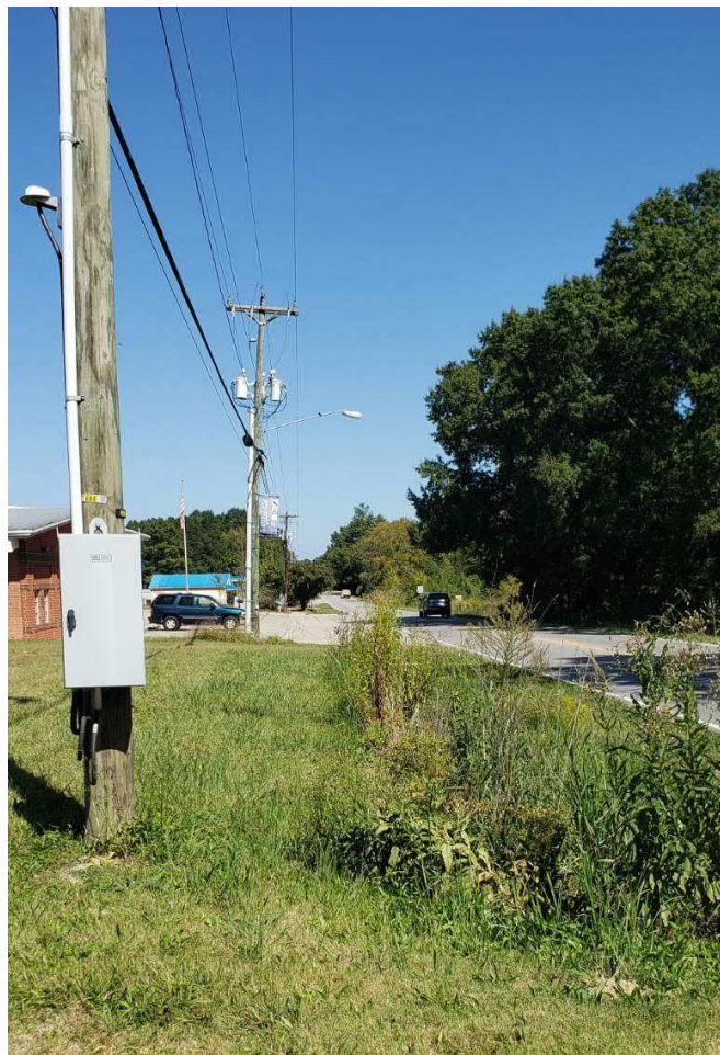
Example of open drainage ditch, vegetation growth, and utility poles that is representative of the majority of the NC 75 and Potter Road right-of-way. This photo is looking east on NC 75 towards the Mineral Springs Volunteer Fire and Rescue.
