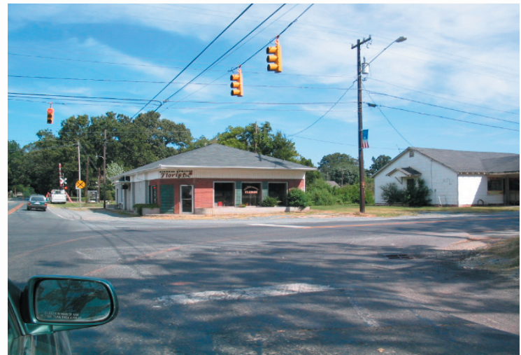
Fig. 57 Existing conditions at main intersection.
