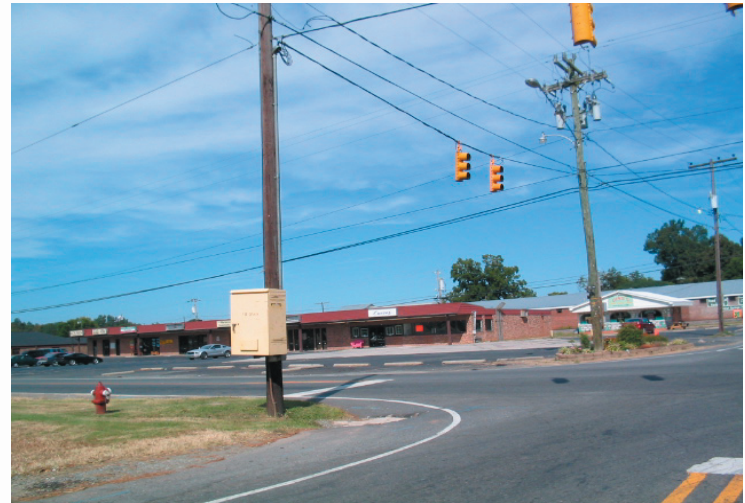
Fig. 59 Existing conditions at main intersection.
