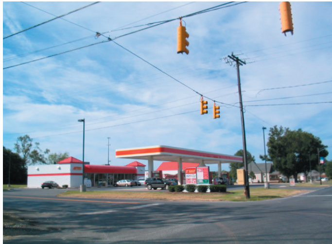
Fig. 58 Existing conditions at main intersection.
