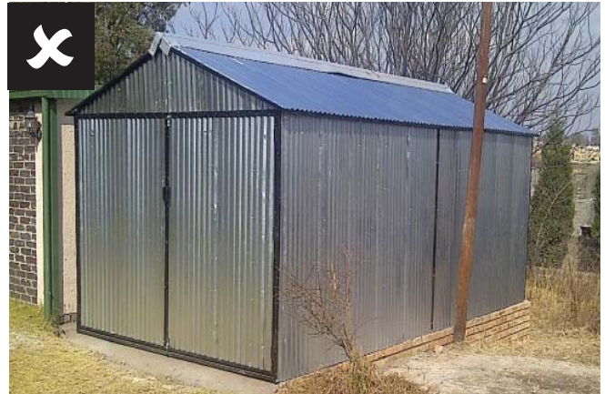
Materials do not match principal structure
