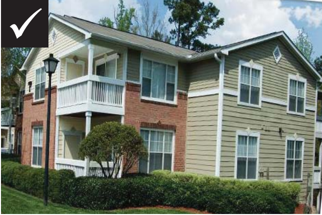
Adequate windows with regular rhythm and alignment
