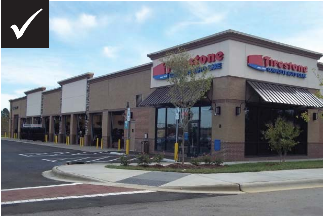
Service bays on secondary building wall
