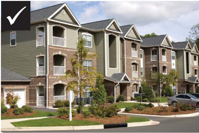
Facade articulation with recesses and projections
