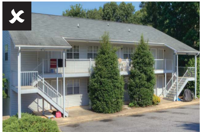
Exterior stairs and circulation corridors
