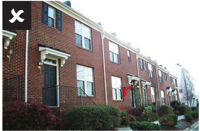
No facade articulation
