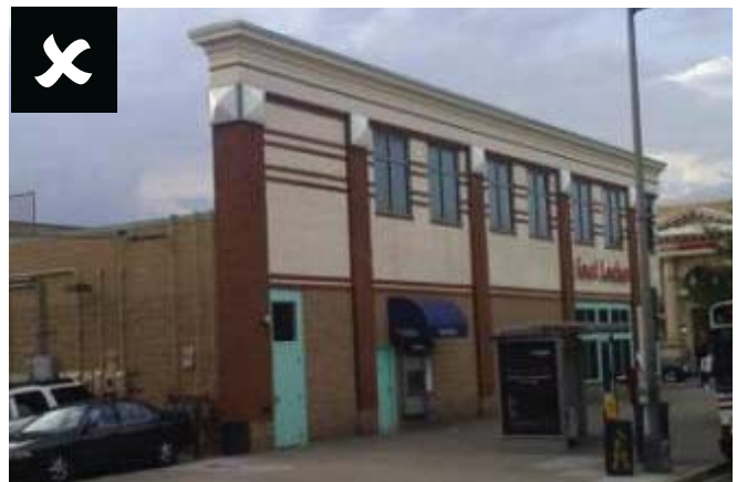
Non-continuous parapet without height changes
