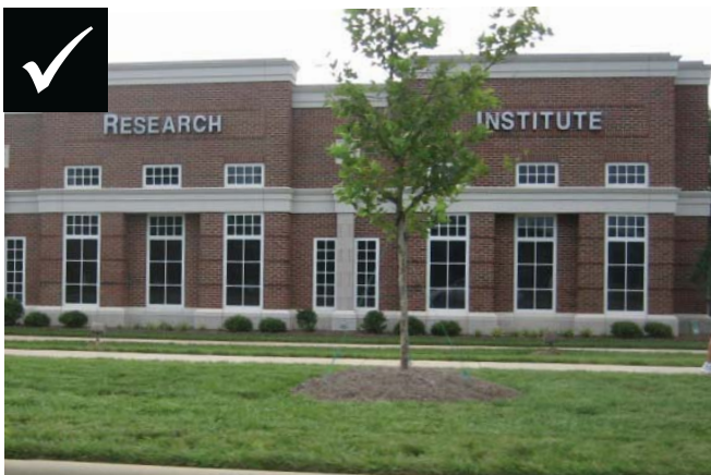
Continuous parapet with height changes
