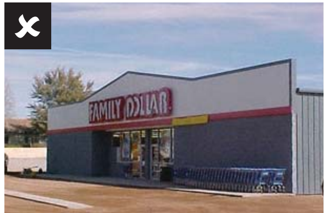
Painted concrete block and metal facades
