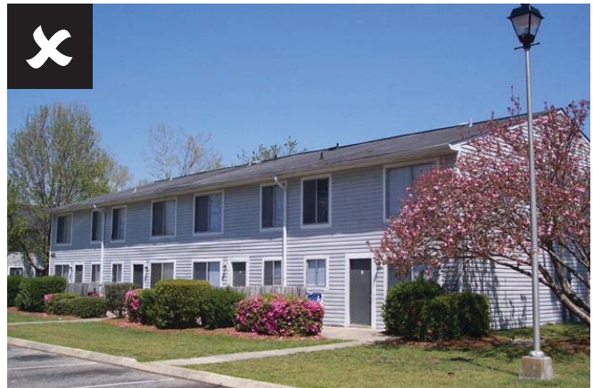
Shallow roof with no variation or side overhang
