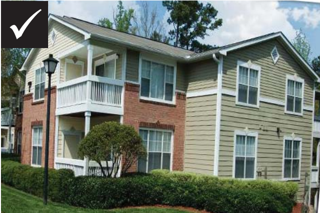
Adequate windows with regular rhythm and alignment
