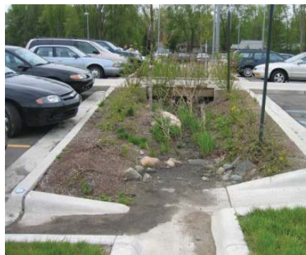
Standard curb and gutter directed into landscaped areas
