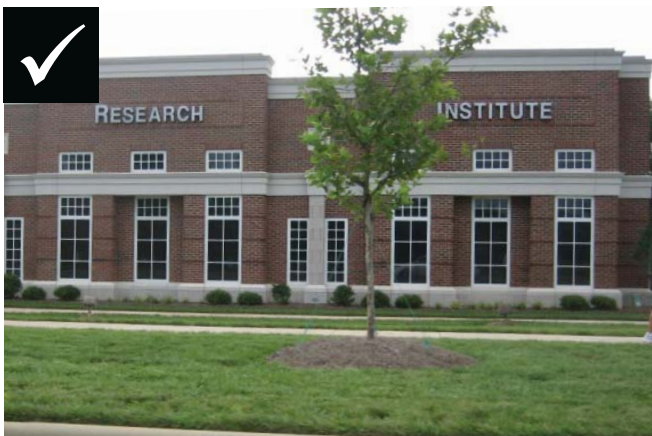
Continuous parapet with height changes
