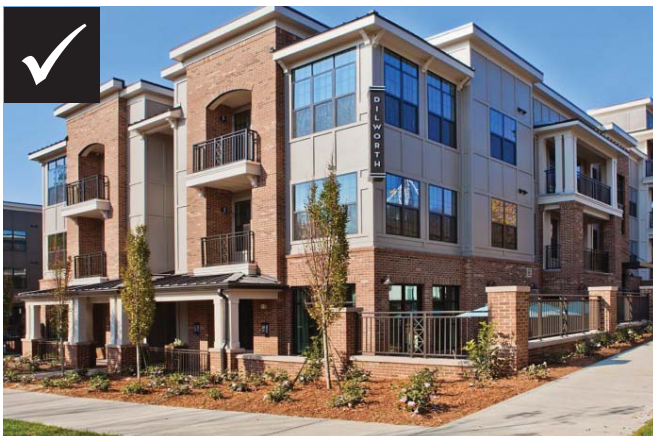
Flat roof with decorative parapet and variation
