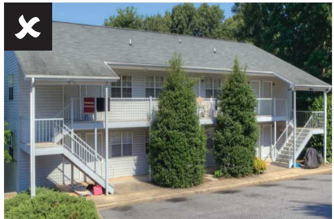
Exterior stairs and circulation corridors
