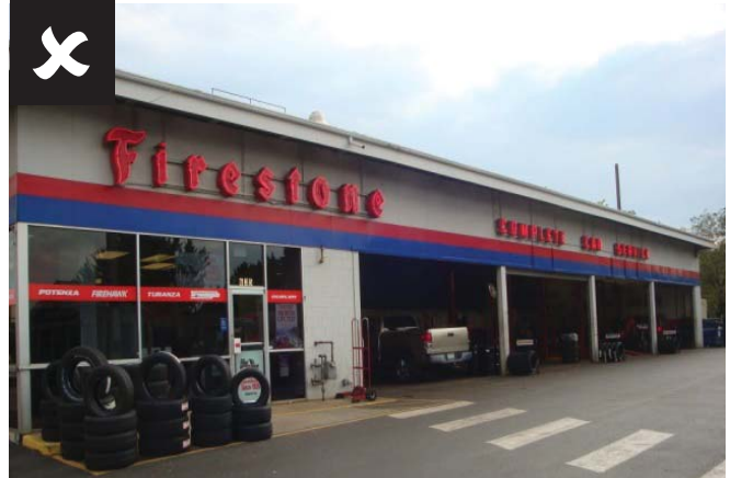
Service bays on primary facade
