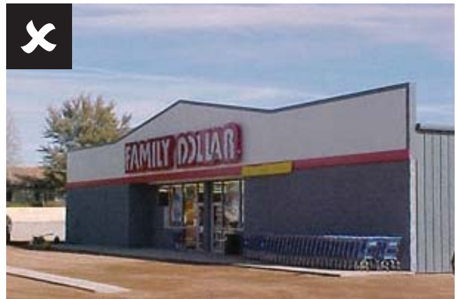
Painted concrete block and metal facades
