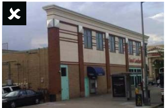
Non-continuous parapet without height changes
