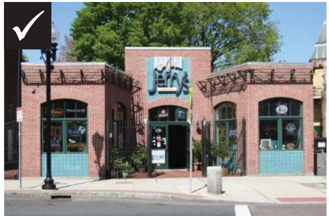
Recessed openings and decorative metalwork
